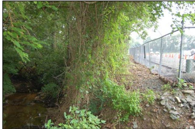
*An example of an inadequate stream buffer between a parking lot and the stream.*
